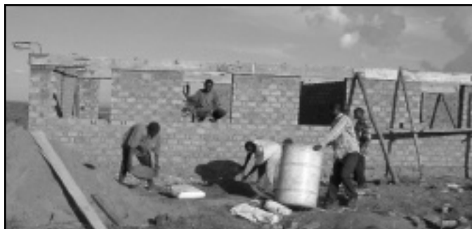
The ECAT under construction in January.
